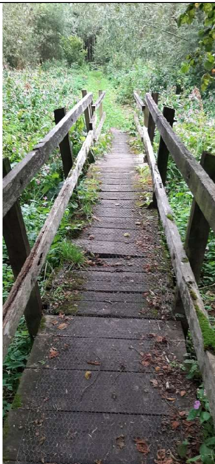
Footbridge – rotten boards (handrails and post, especially on LHS)
